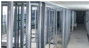
Drywall tracks to concrete and steel
