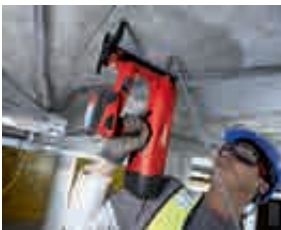
Threaded rod attachments to concrete
